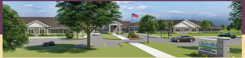
Currently under construction at 350 South Marketplace Blvd. in Lansing, MI
