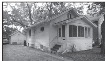
Property 3313 - Lansing Illinois Ave.
