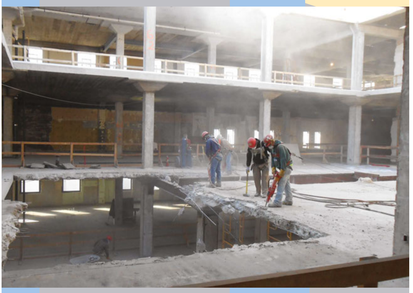
Courtesy Granger Construction
